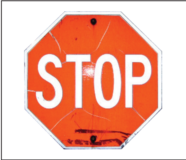
The red background of this stop sign has many cracks due to environmental factors.
