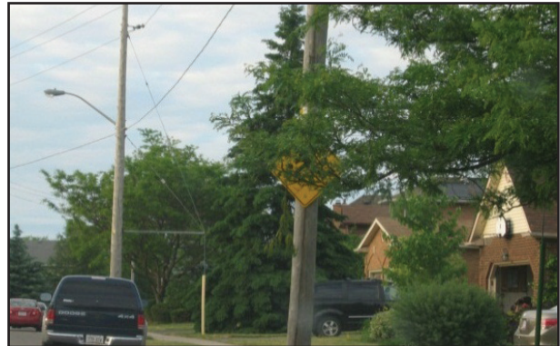
Vegetation control maintenance required.
